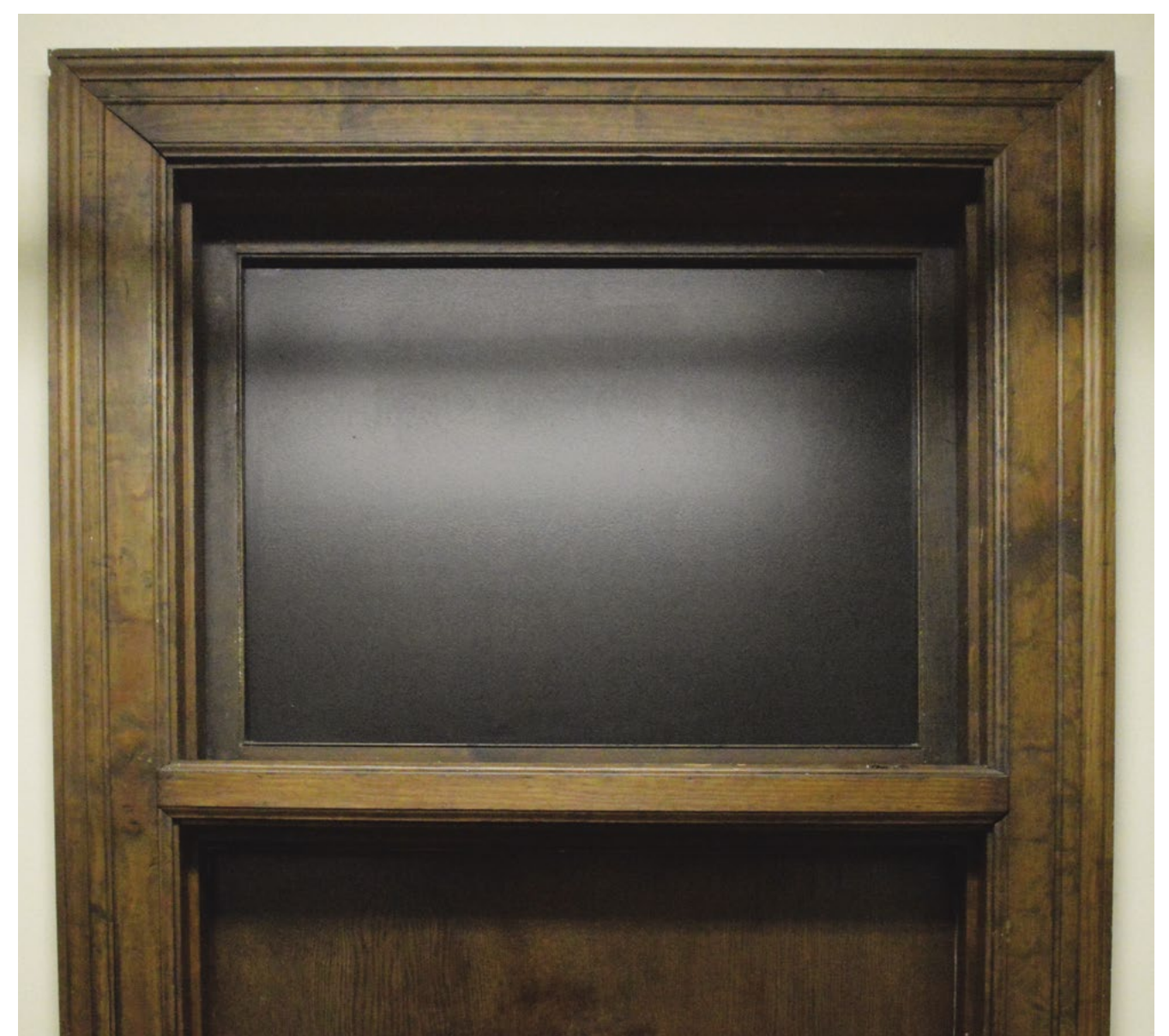
Using a metal crank on the bedroom side, this transom or window above the door could be opened for ventilation and provided light to the hallway from the windows on the outside walls.
