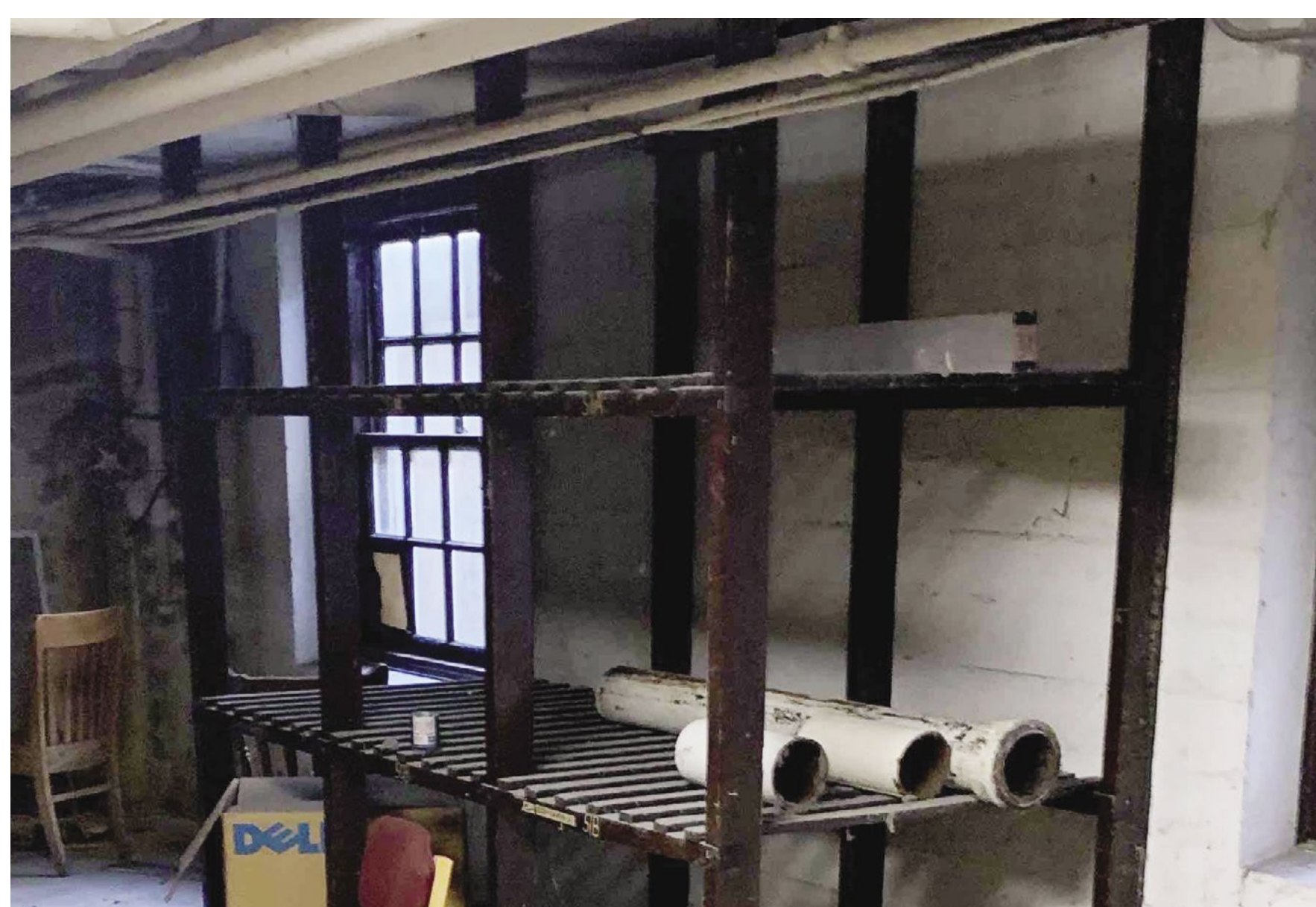
Pre-demolition image of trunk storage racks, 2019.
